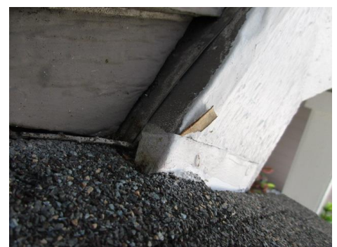
Flashing with reversed lap
