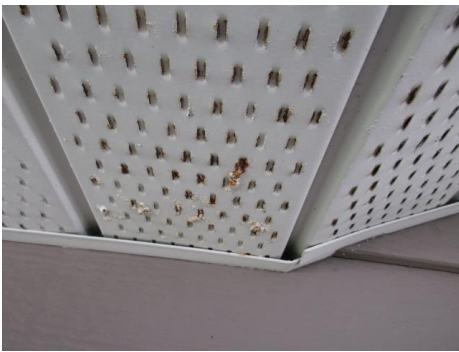
Corrosion under cut drip edge
